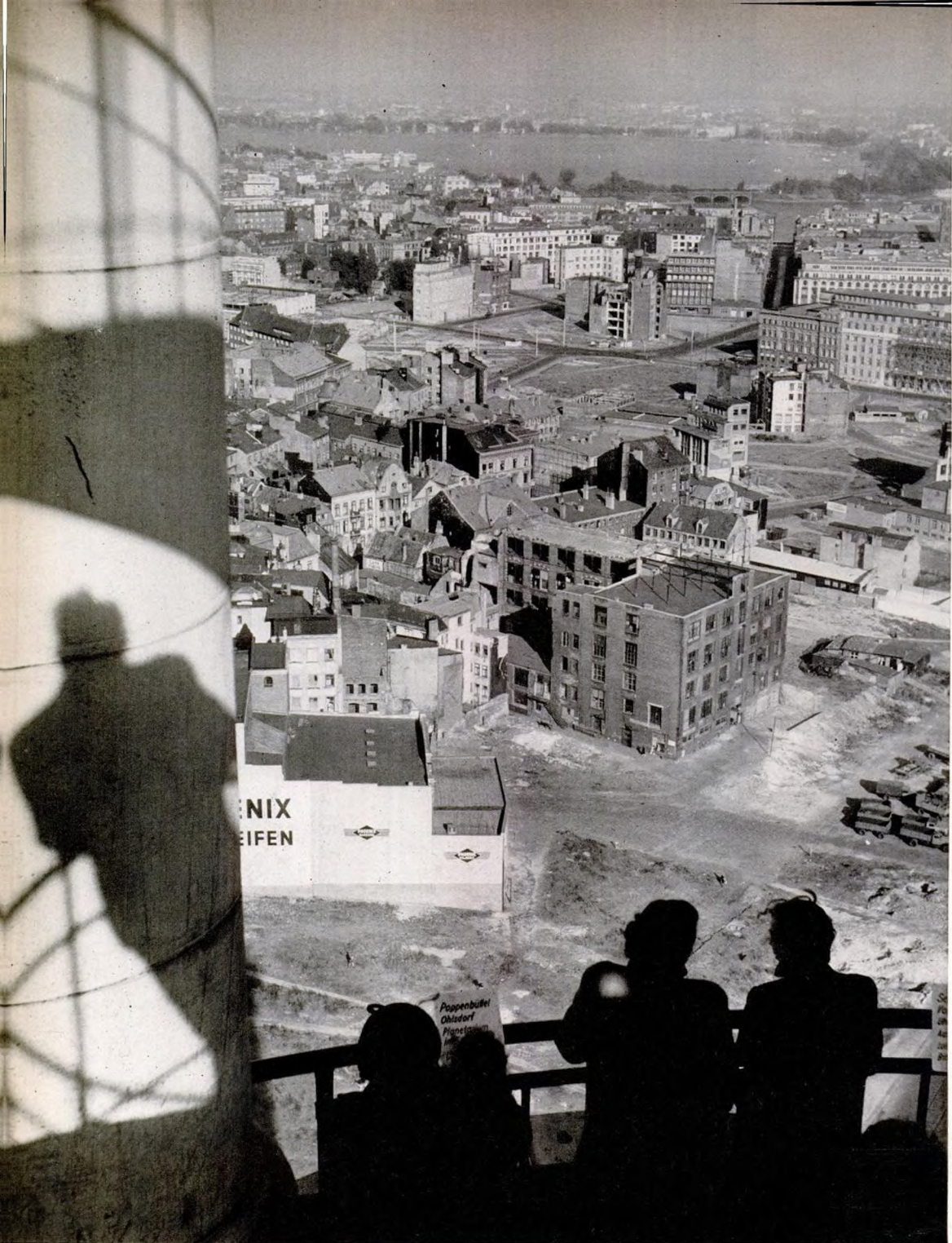
SIGHTSEERS' VIEW from the 433-foot bell tower of St. Michael's Church, the highest point in Hamburg, looks across a vast area of mixed destruction and rebuilding and shows how well the city has cleared away rubble both to make way
